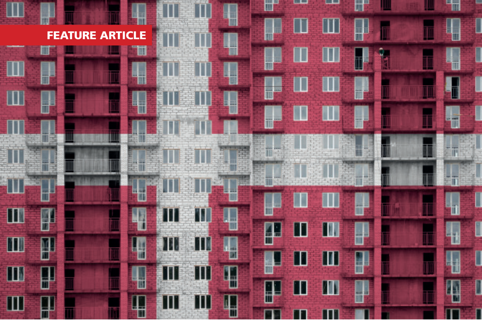
Denmark flag depicted in paint colours on multi-storey residential building under construction. Credit: Mehaniq/Shutterstock
